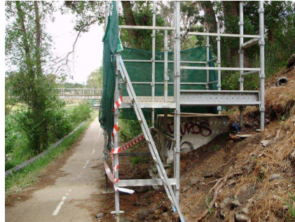
Erection of scaffolding and work platforms above raised manholes was necessary
